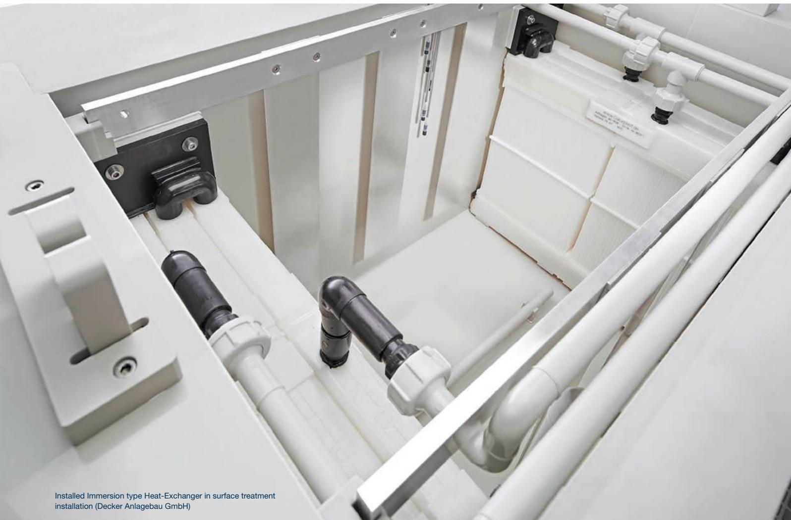
Installed Immersion type Heat-Exchanger in surface treatment installation (Decker Anlagebau GmbH)
